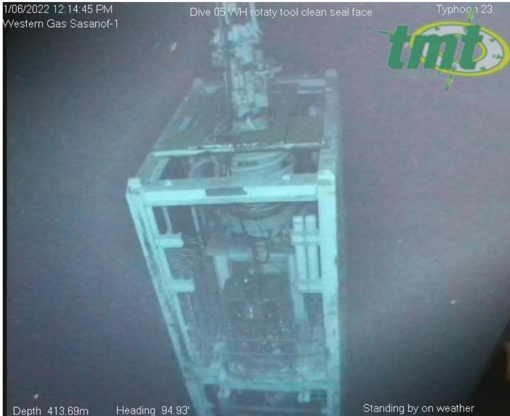
*Blow out preventer being deployed in open water.*
